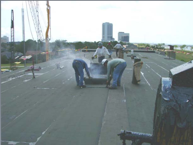
Workers install a new roof at the Bonnabel Pump Station in Jefferson Parish.
